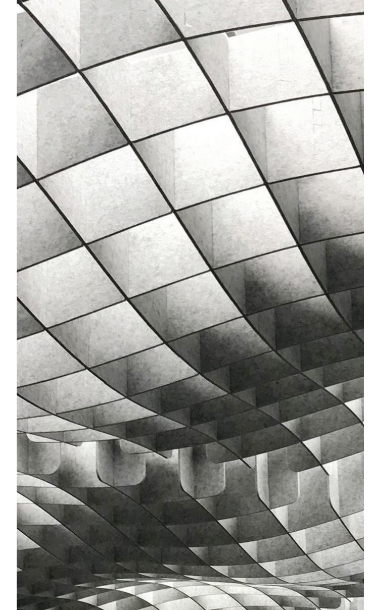
EzoBord Acoustical Net canopies are completely customizable, add flow, color and acoustical balance to open ceiling environments while reducing unwanted noise.
