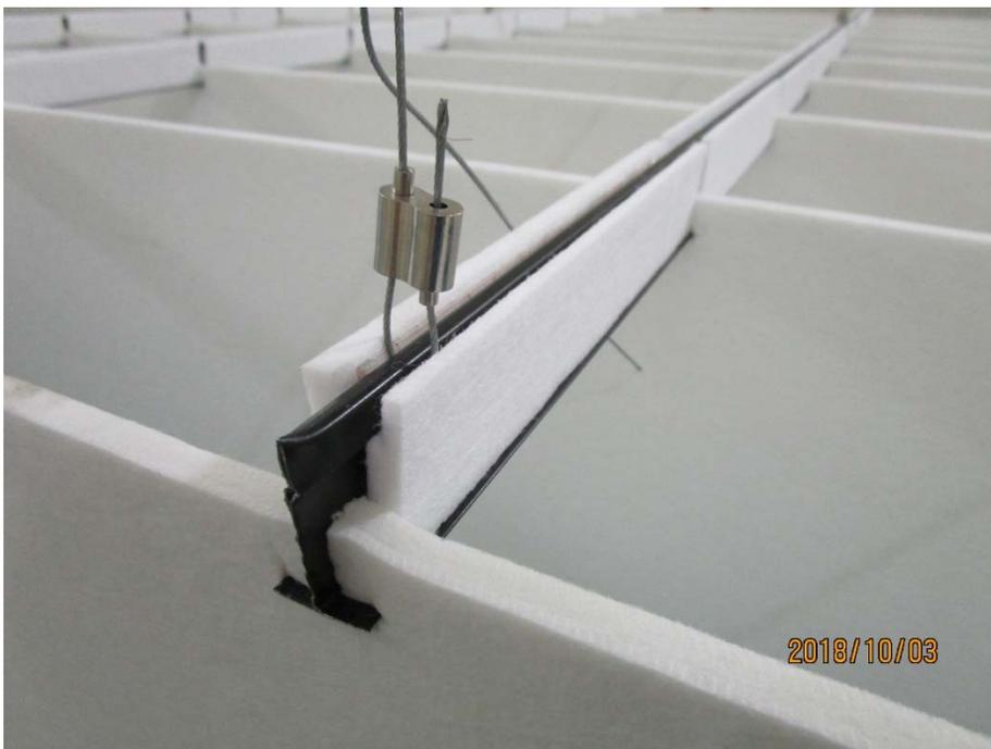
Figure 2 - Detail of baffle material, spacers, mounting method
