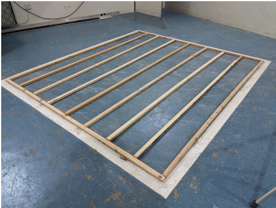
Figure 2 – Wood furring spacers in test chamber prior to installation of test specimen
