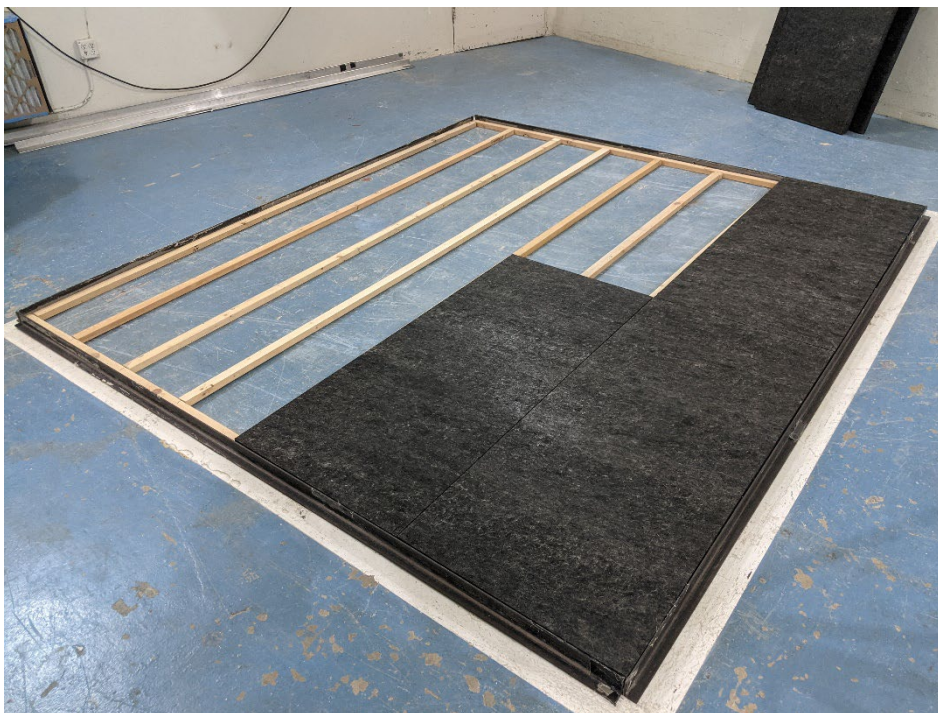
Figure 4 – Specimen partially installed over spacers
